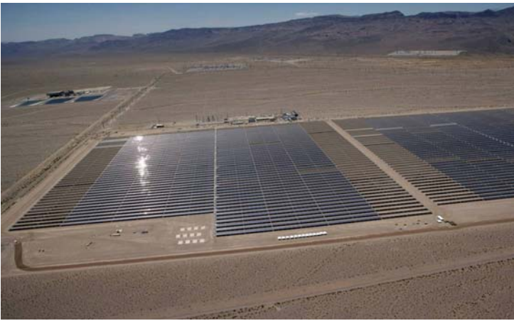
Figure 5: 64 MW Nevada Solar 1 Solar Plant
