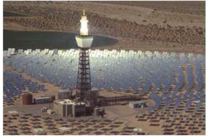
Figure 8: 10 MW power tower pilot project, Barstow, CA
