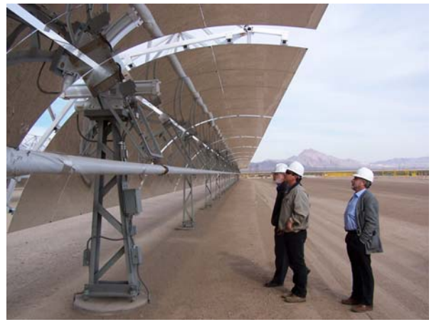
Figure 6, Nevada Solar 1 solar collector
